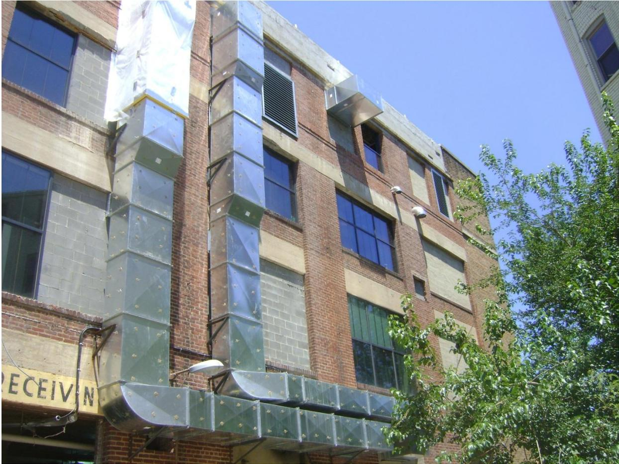
Figure 36: Mechanical Ductwork on Exterior Facade, Picture Taken by Clara Watson
